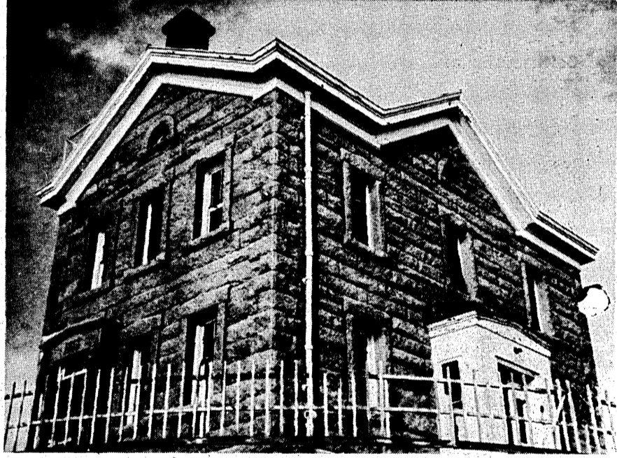
The county acquired something very special when it took over the Cedar Point Lighthouse overlooking Gardiner's Bay in 1969.
